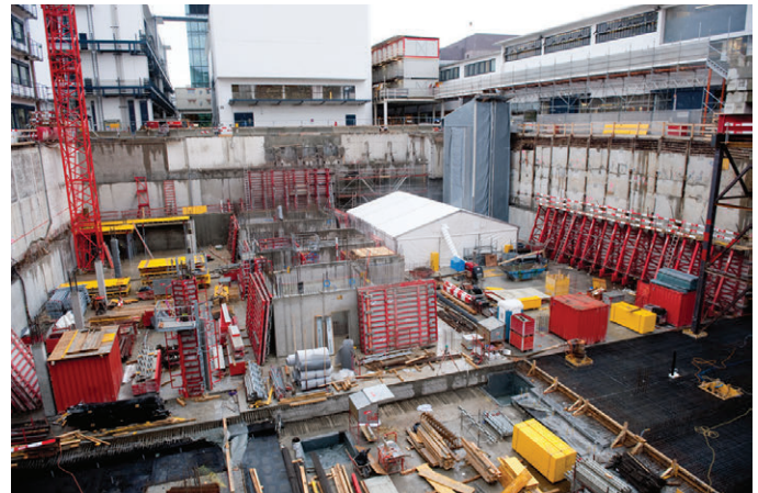
Finished construction pit in a very tight construction area.
