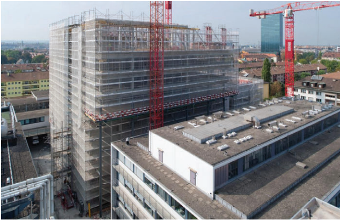
Civil phase nearing completion 2009.
